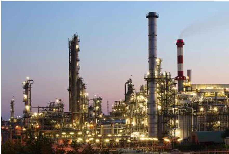
Fig. (1). Picture of the Zawia refinery site in Libya
